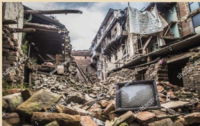
Gambar 2. Kerusakan Akibat Gempa Bumi (sumber: https://www.shutterstock.com/image-photo )
